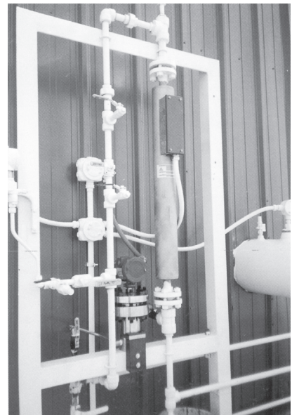
Typical installation. Note how the transducer is rigidly clamped, isolation valves are provided for easy maintenance.
